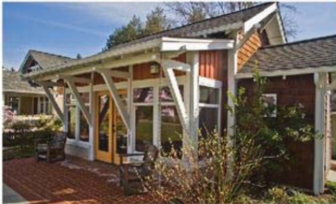
Commons with large overhangs is welcoming
