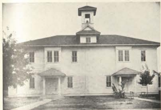
SCHOOL HOUSE IN DISTRICT NO. 46, ROSWELL, IDAHO.
