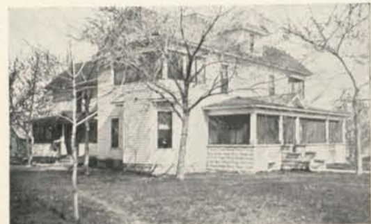
RESIDENCE OF A. J. ROCKWOOD, ROSWELL, IDAHO.
